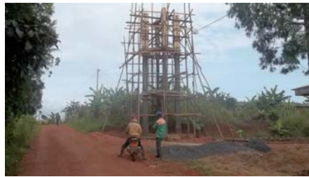
4.suite armature des 4 poteaux
